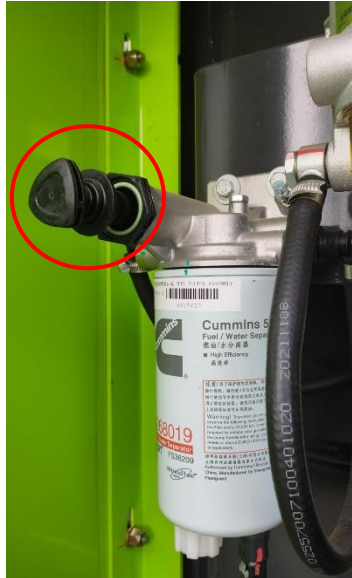
Figure 5-20. manual pump for fuel filter
